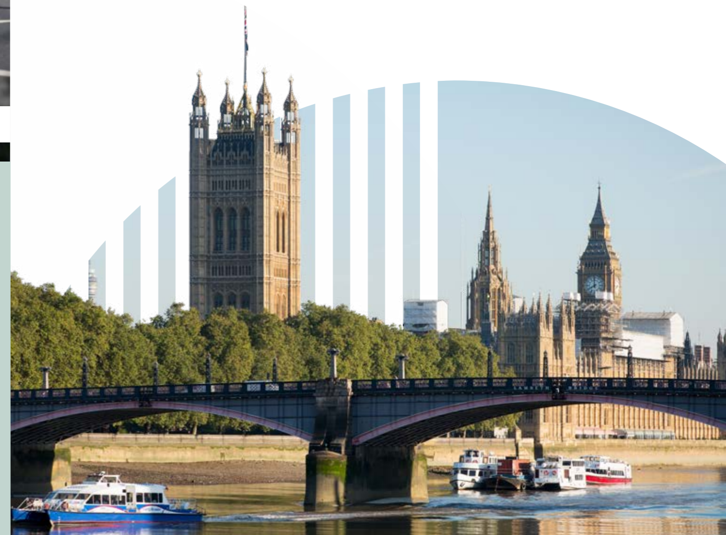
We will improve Lambeth Bridge and make it safer
